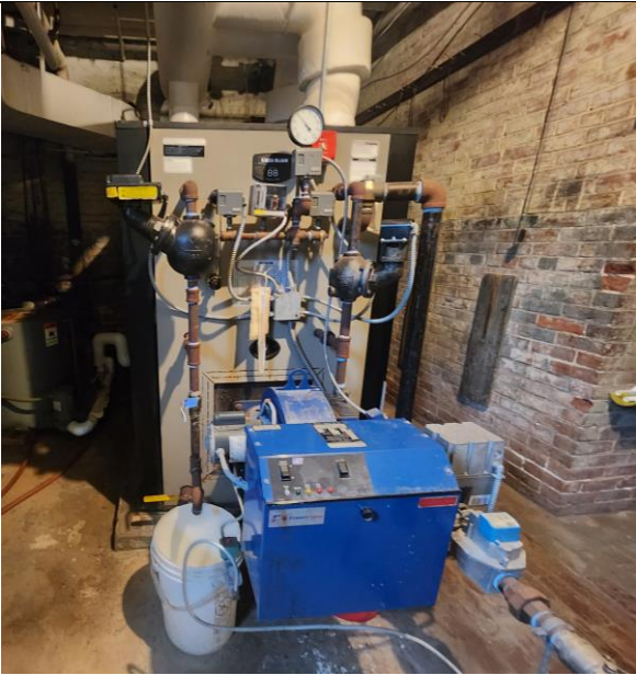
Weil McLain Boiler and Power Flame Burner
