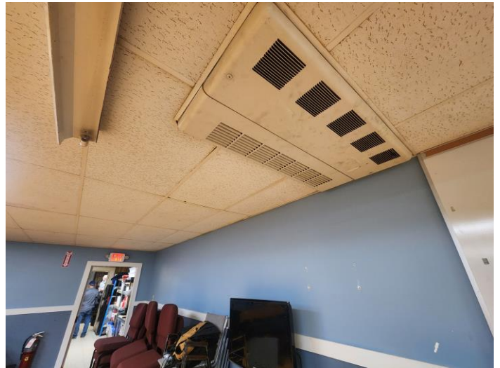
Hot water cabinet unit heaters
