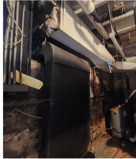
Boiler combustion air and FCU outside air intake
