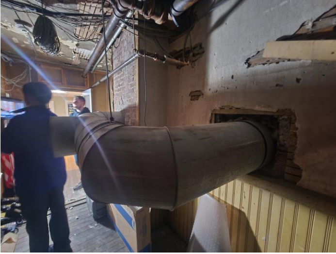
Existing Boiler flue
