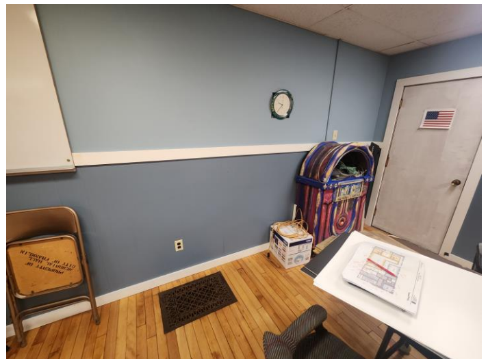
Abandoned Floor grilles for old steam system
