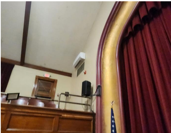
Auditorium Cooling and fresh air supply grille
