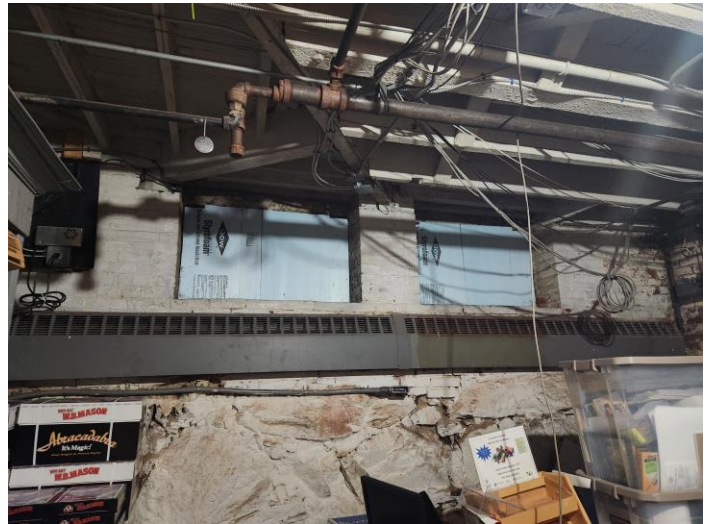
Typical Fin tube in storage areas of basement and uninsulated hot water piping
