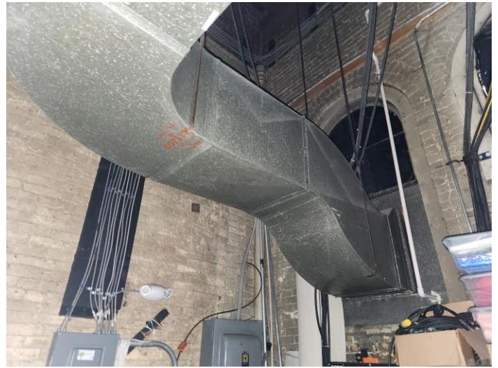
Auditorium AHU fresh air connection above door
