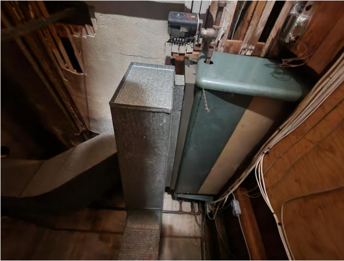
Hot water fan coil unit
