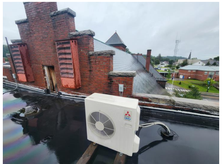
Auditorium condensing units on roof
