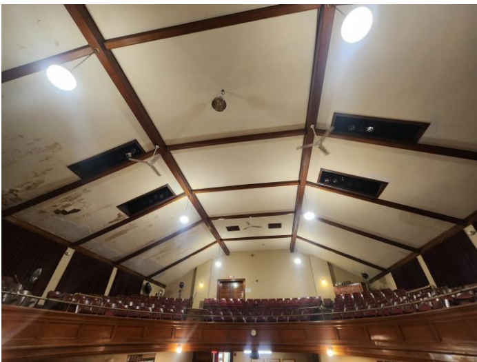
Auditorium ceiling with destratification fans
