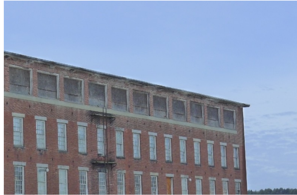
6 Mill #1 - North Elevation - detail at upper floors showing modified windows at top floor
