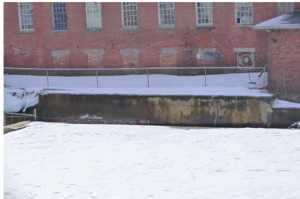
10 | Mill #2 - North Elevation - detail at lower level showing infilled windows
