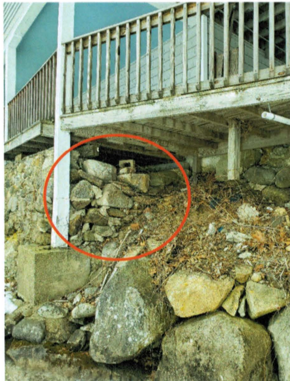
Figure 2: Loose wall to be reset with mortar, foundations of support posts to be replaced.
