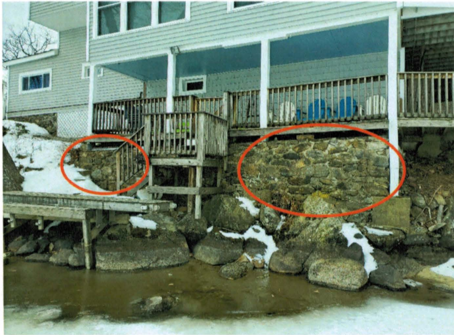
Figure 1: Stone retaining wall to remain and be repointed as necessary. Landing, steps to dock and dock to be removed and replaced in existing location.
