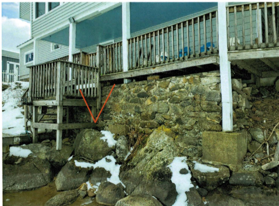
Figure 3: Area of wall to be resurfaced.
