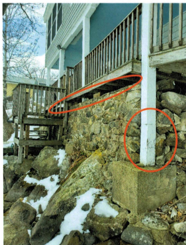
Figure 4: Concrete cap to be installed and timber post repaired.
